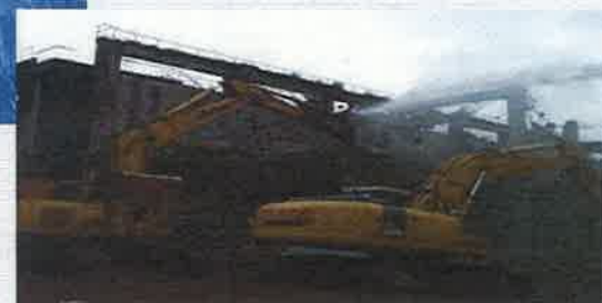
裸露處加強灑水降低揚塵逸散
