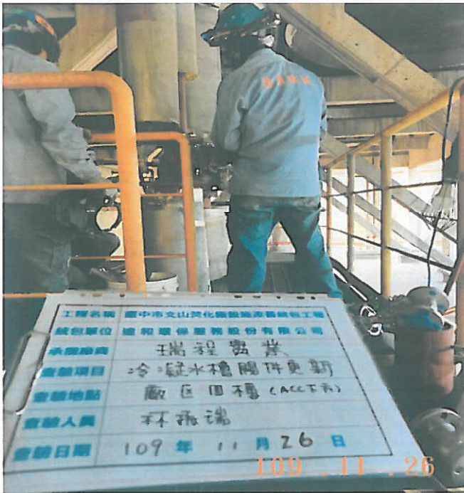
舊品閥件拆卸
